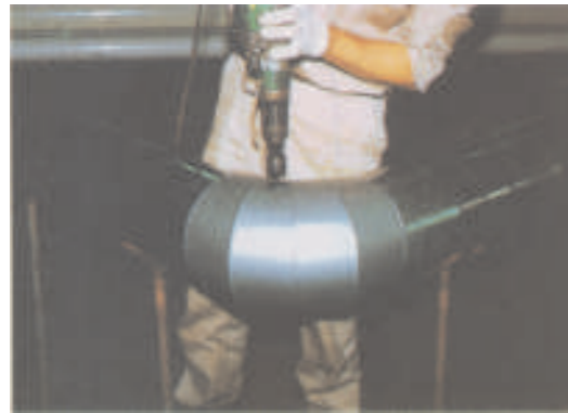
Open pour-hole on fitting cover
