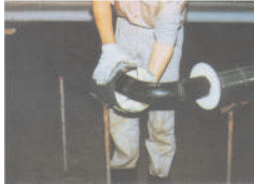
Place sleeve in position
